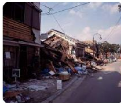
iStock 100+ After Earthquake Kobe Japan
