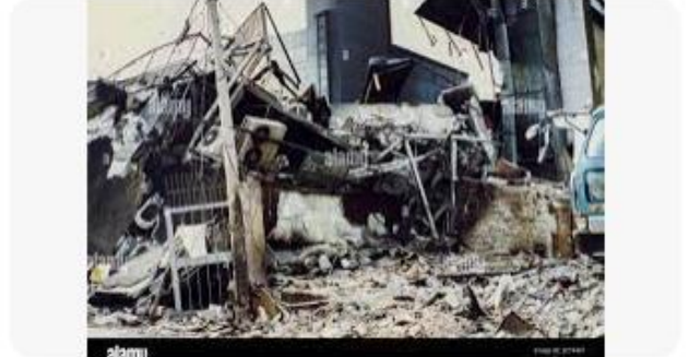
Alamy Hanshin awaji earthquake hi-res stock photograph...
