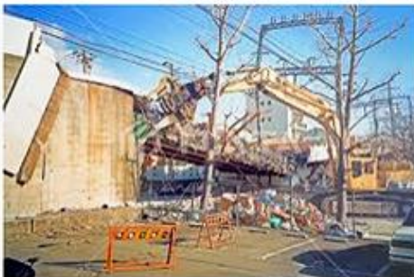
PIXTA Hanshin Awaji Earthquake restoration work # 2 - Stock Photo
