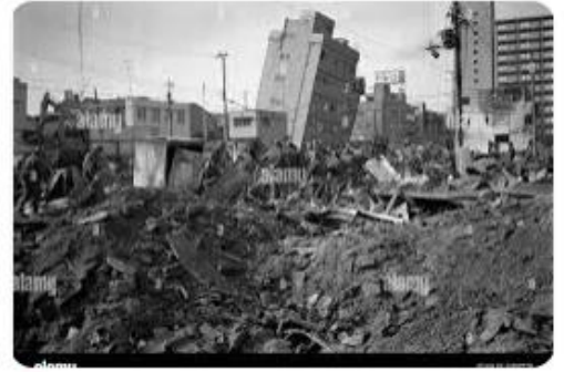
Alamy Hanshin awaji earthquake hi-res stock ...
