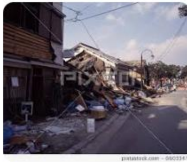
PIXTA House collapsed Hanshin Aw...
