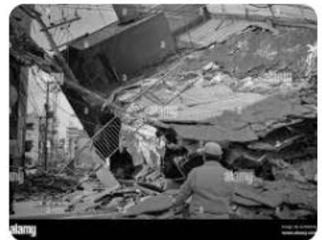
Alamy Man stops and looks upon collapsed structure
