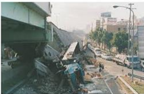
Timenote Great Hanshin earthquake
