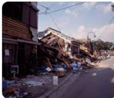
iStock 100+ After Earthquake Kobe Japan
