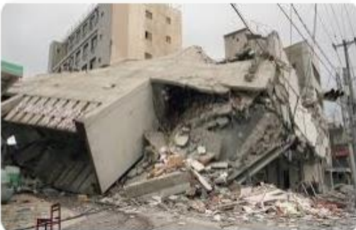
Reddit The building which collapsed in the afte...
